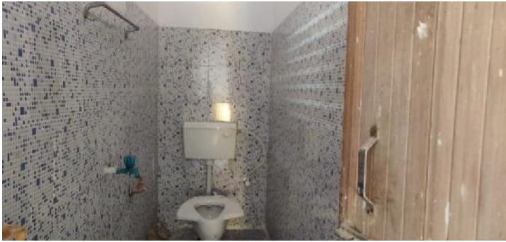
Renovated toilet at Baidyapara High School.
