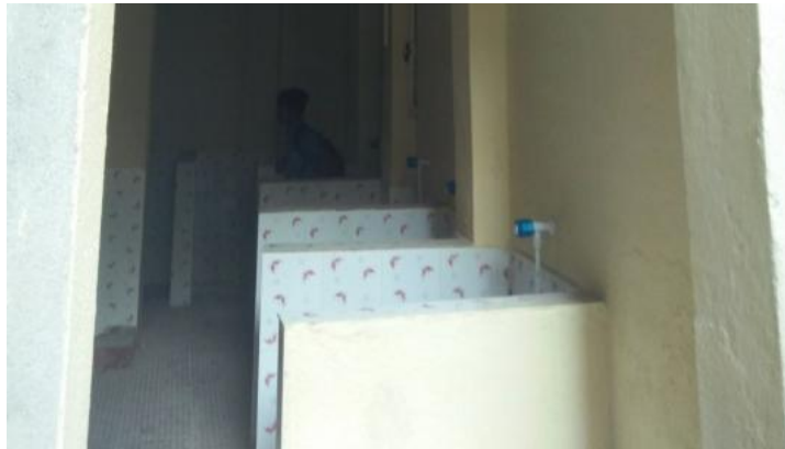
Renovated toilet at St Joseph Primary School, Behala.
